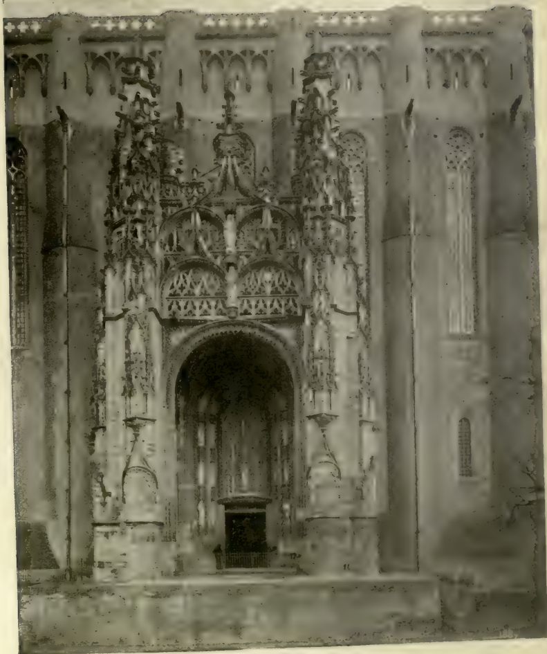
SOUTH PORCH AND SIDE OF NAVE Cathedral, Albi
